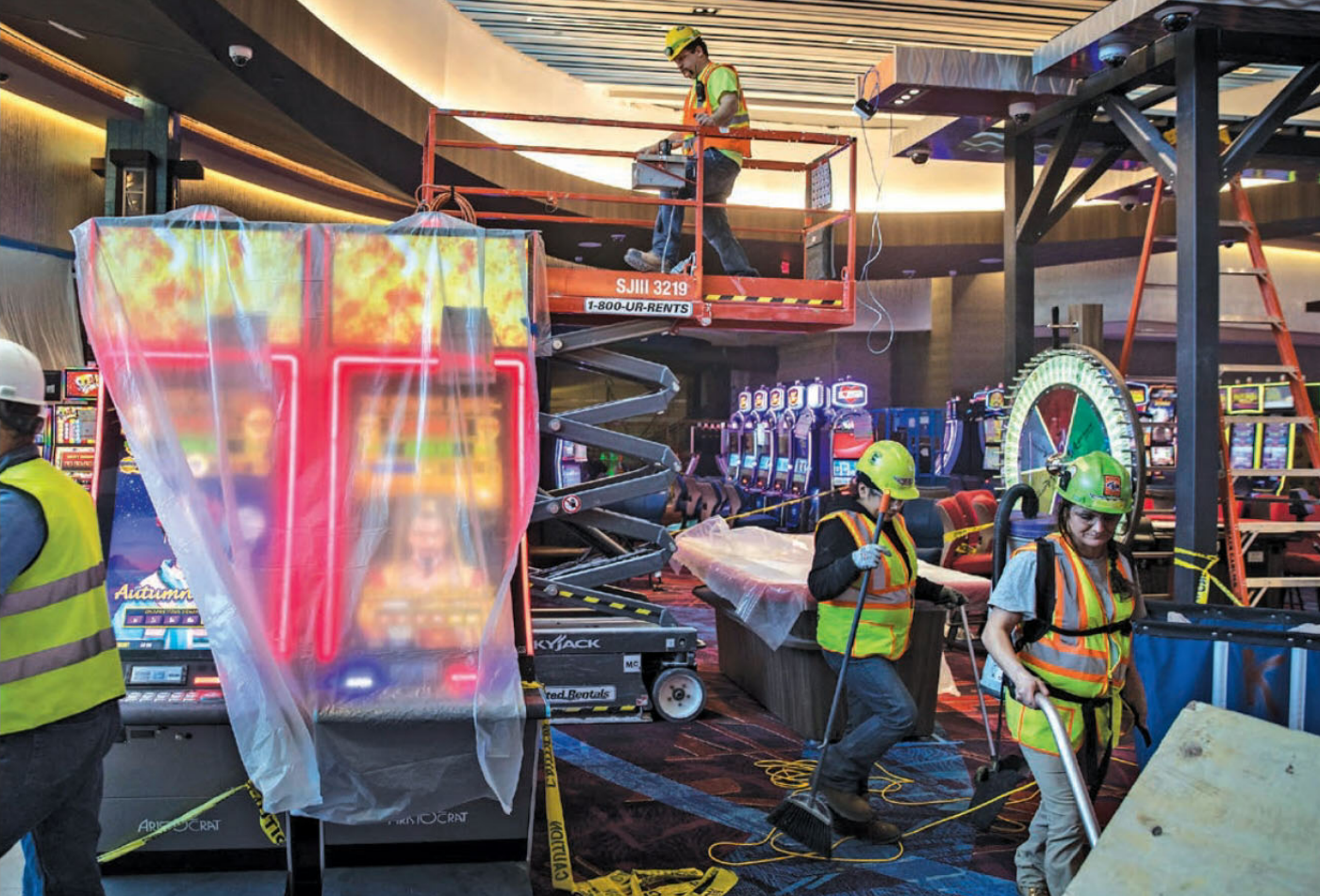
▲ Workers readying Resorts World Catskills for its February opening
